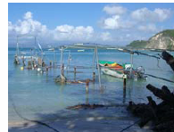
Destroyed berth, Petit Havre
